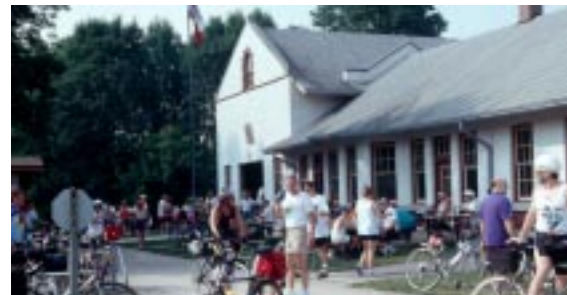
Restored depot at Center Point
