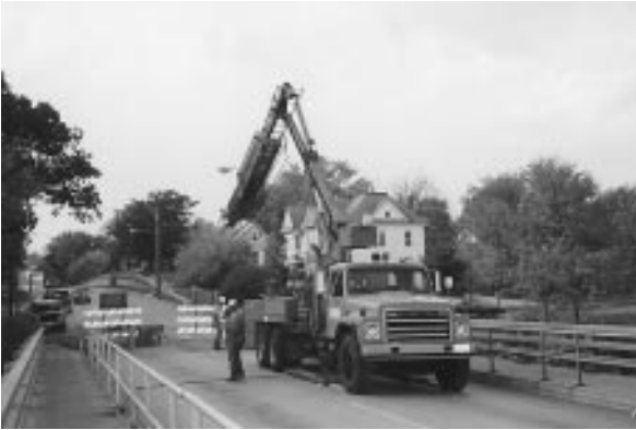
Temporary closure to traffic.
